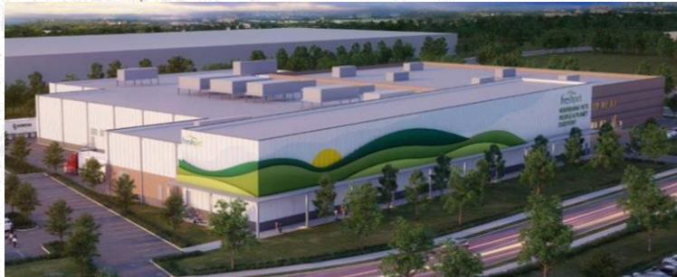
Completed construction and started up Kitchens 2.0 – despite limitations imposed by COVID
